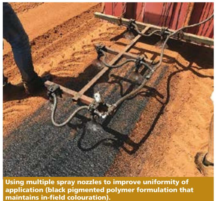
**Using multiple spray nozzles to improve uniformity of application (black pigmented polymer formulation that maintains in-field colouration).**
