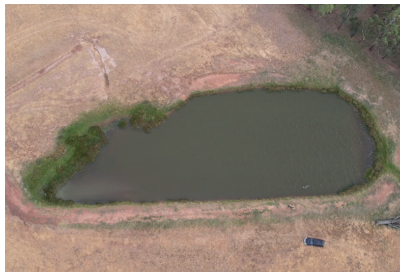
A droneshot of the Dookie control dam.
