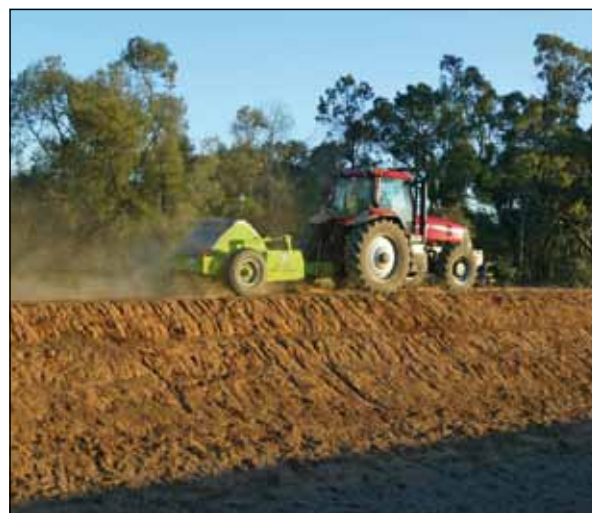
An impact roller working on a channel bank.
