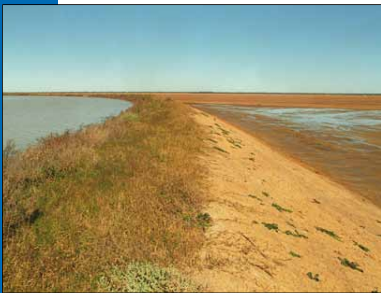
Compaction is often a viable option to minimise water loss.
