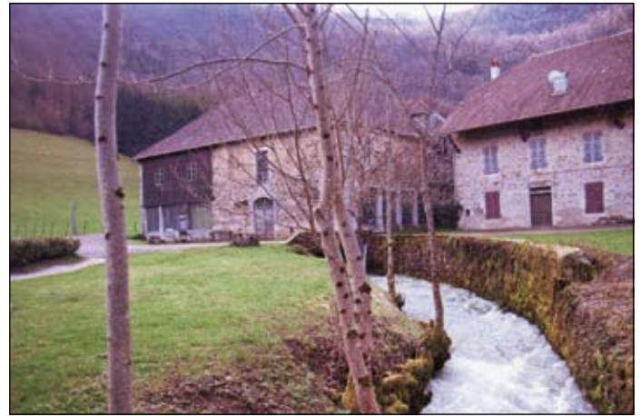
Pictured is the canal tributary, excavated 200 years ago, which passes under La Taillanderie and provides power to the giant water wheels within the factory. (Photo IMJ)
