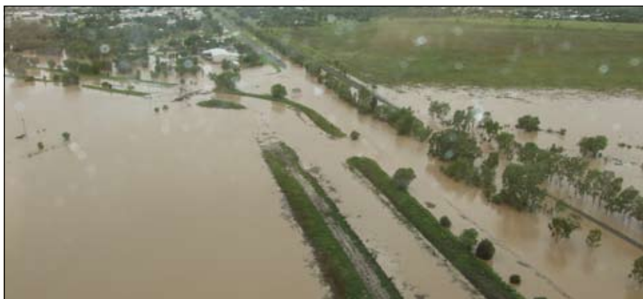
The main bridge and railway line into Emerald.
