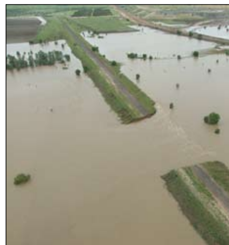
Levy banks were breached in many cases.
