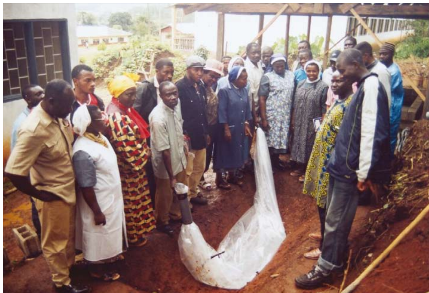
Biogas course participants instal a small demonstration poly plug-flow digester at the National Polytechnic in Bamenda, capital of North-West Province in Cameroon.
