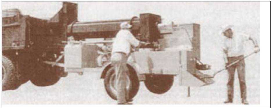
The Wylie was usually towed behind a tip truck, which carried the supply of aggregate (blue metal).
