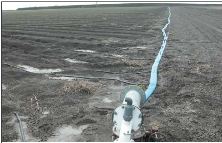
A drip system installation on the Darling Downs.
