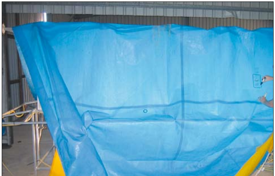
Performing yearly tarp maintenance.
