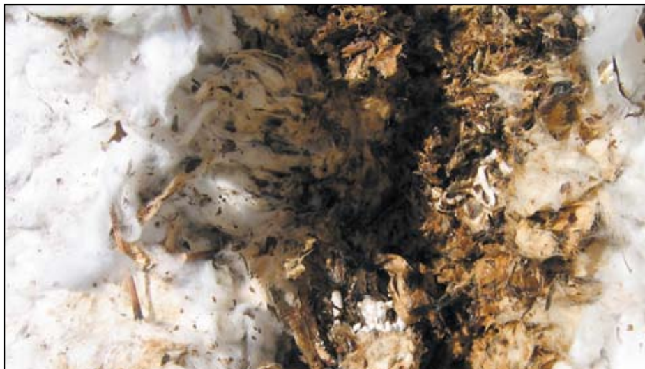
A weather damaged module — complete with mushrooms.
