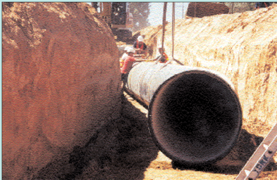
Open channels were replaced with pipes.
