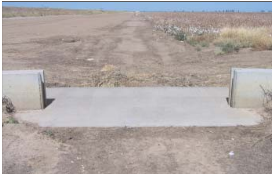
These channel checks are large enough to drive machinery through, making channel maintenance easier. This particular bankless channel is 3.8 km long.
