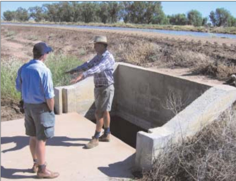
Large capacity structures are a part of bankless channels.
