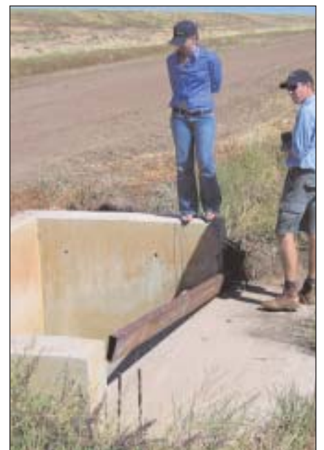
Negligible amounts of tailwater leave the field, but the higher capacity for storm events remains.
