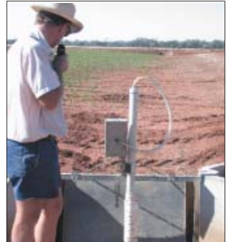
Automation is readily available to allow the doors to open at a set depth, simplifying the irrigation process. This unit is portable to other culverts.
