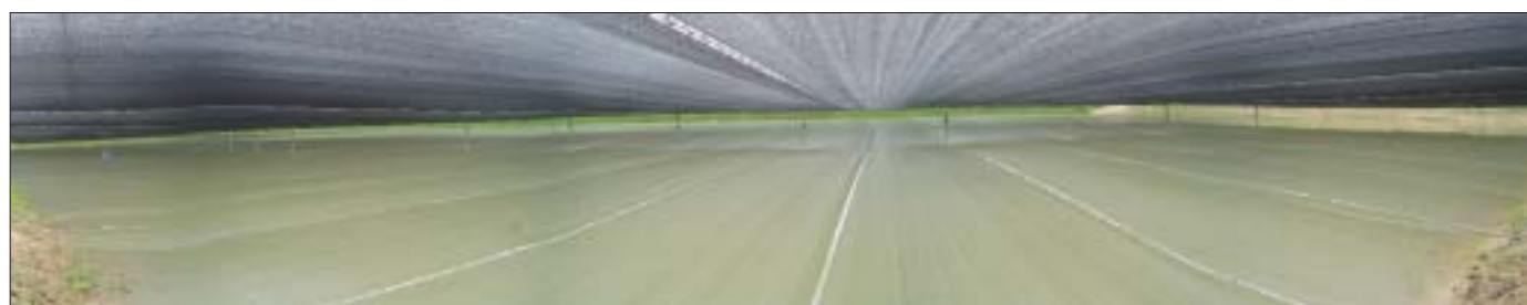
Netpro shade cloth structure reduces evaporation by around 75 per cent.
