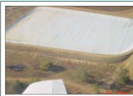
Aerial shot of the Evaporation Control Systems E-VapCap floating cover at Moonrocks Farm, St George.
