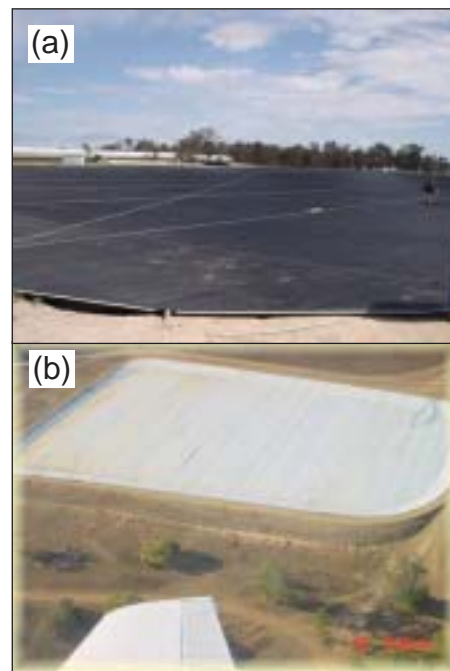
Evaporation management trial sites: Netpro shade structure (a); and E-VapCap cover (b).
