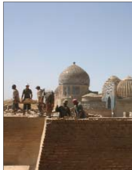
Mosque repairs underway in Samarkand.
