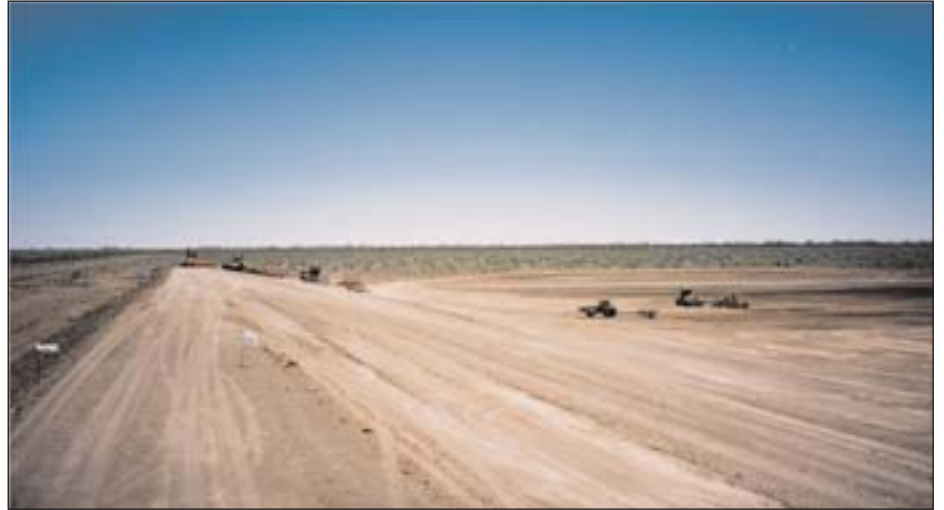
At “Cavillon” Dirranbandi, raising a dam wall during the drought.
