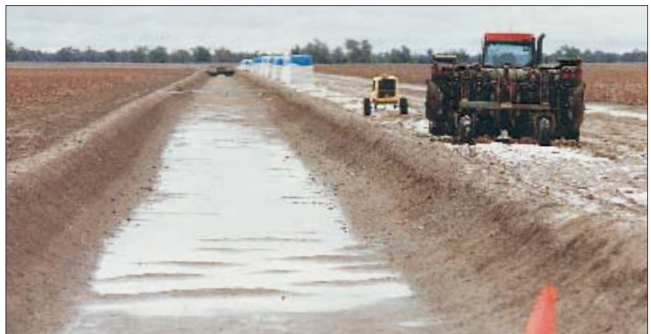
Channels should be positioned in areas with low risk of excessive deep drainage.
