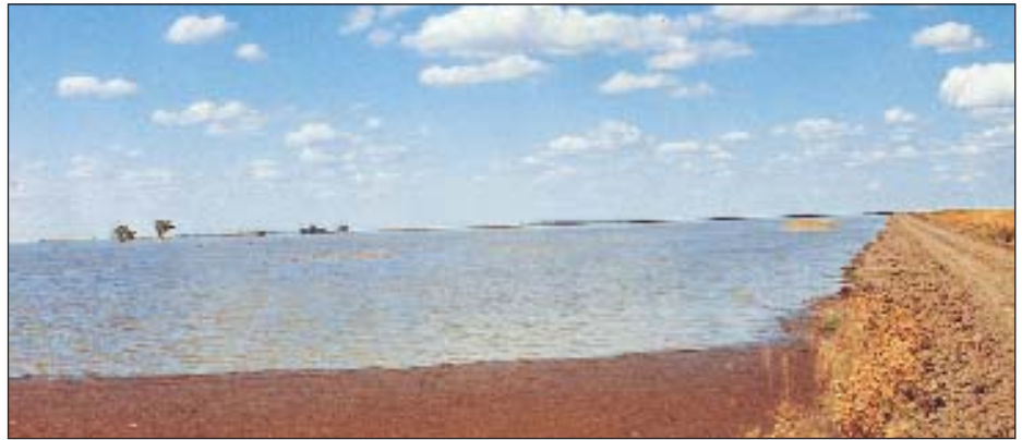
Some storages have been sited in unsuitable areas.
