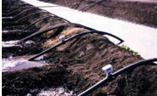
Once initialised, the metered siphons are started and stopped as per normal.
