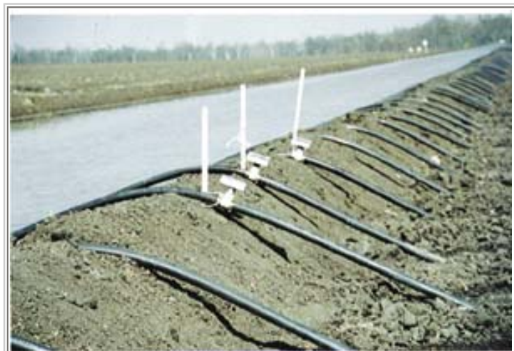
GLI flow sensor with the Irrimate logger measuring siphon flows.
