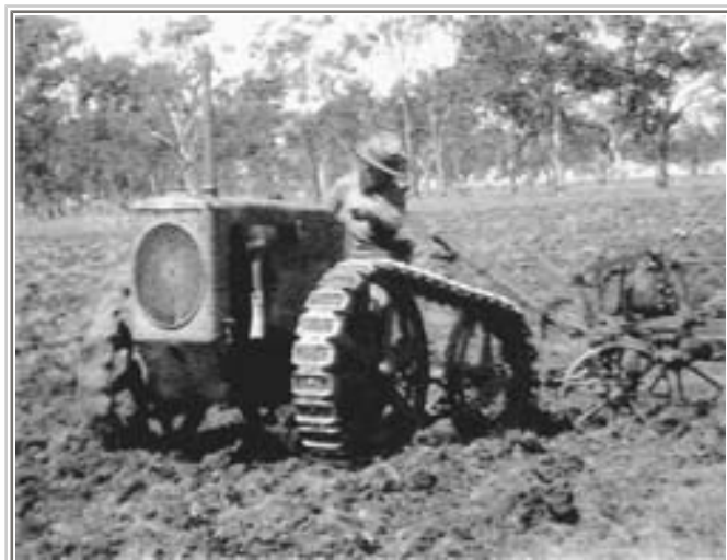
A historic photo taken in 1925 of a German imported Stock crawler tractor featuring front drive. The demonstration took place somewhere in Victoria and is interesting because it was the first front drive crawler ever seen in Australia. The concept was re-invented by Ransomes in the 1930s. (Photo from IMJ archives.)
